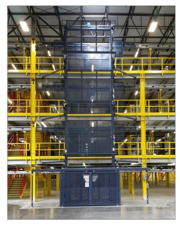
Guide columns are 6" wide flange sections. The carriage is fabricated of 4" or 6" structural members with a steel deck plate. Additional deck surfaces are available.
